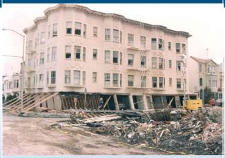
Seismic Evaluation and Retrofit Of Multi-Unit Wood-Frame Buildings With Weak First Stories
